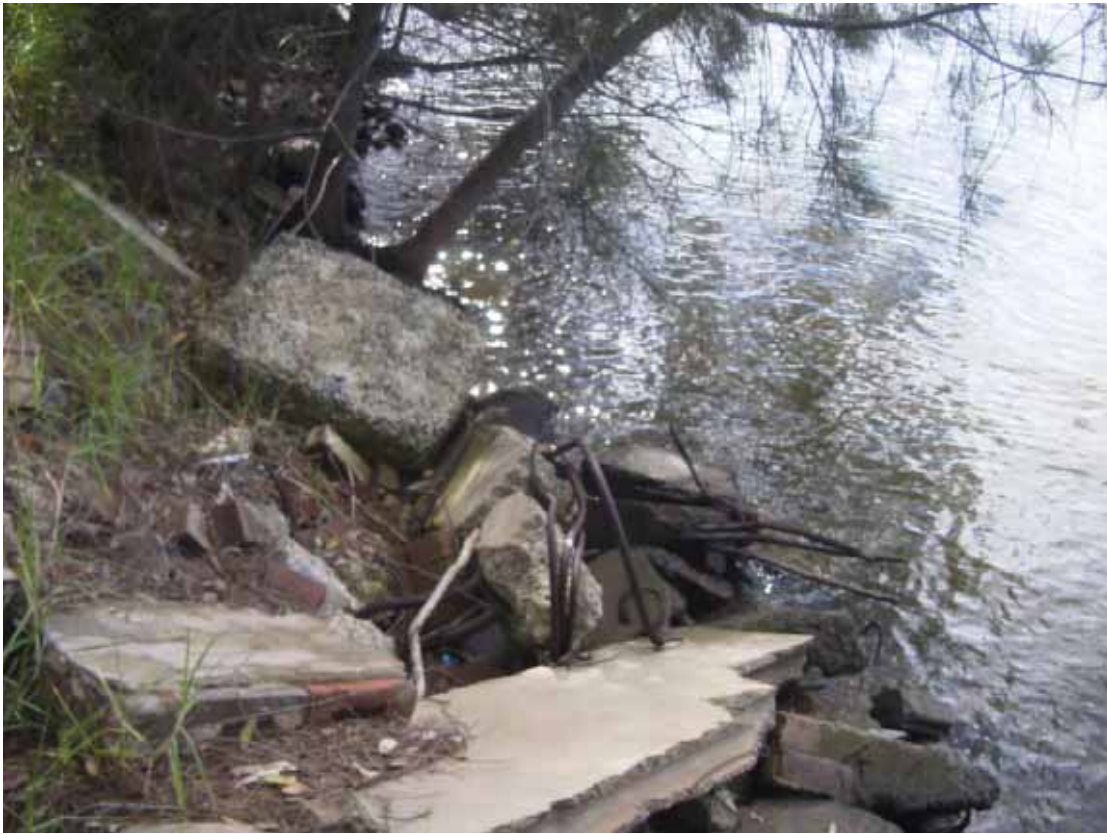
Figure 30. Masonry and concrete fill material.
