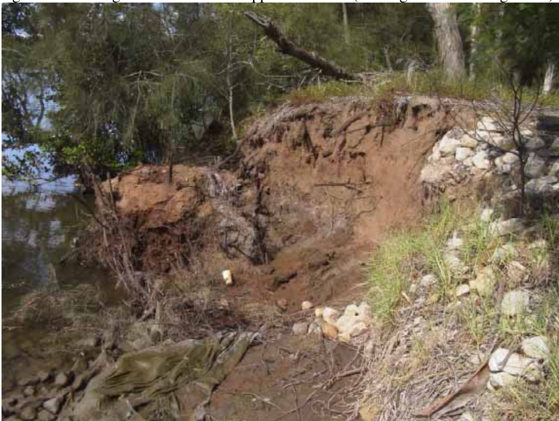
Figure 25. Detail of active bank erosion including exposure of silt-cloth plus slumped rubble fill treatment (looking south from Figure 23).
